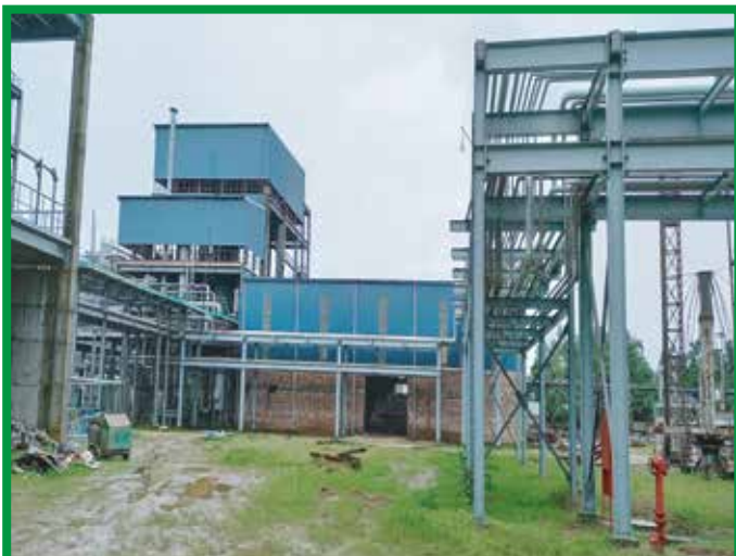
SR Chemical Industries Ltd., Serajganj.
