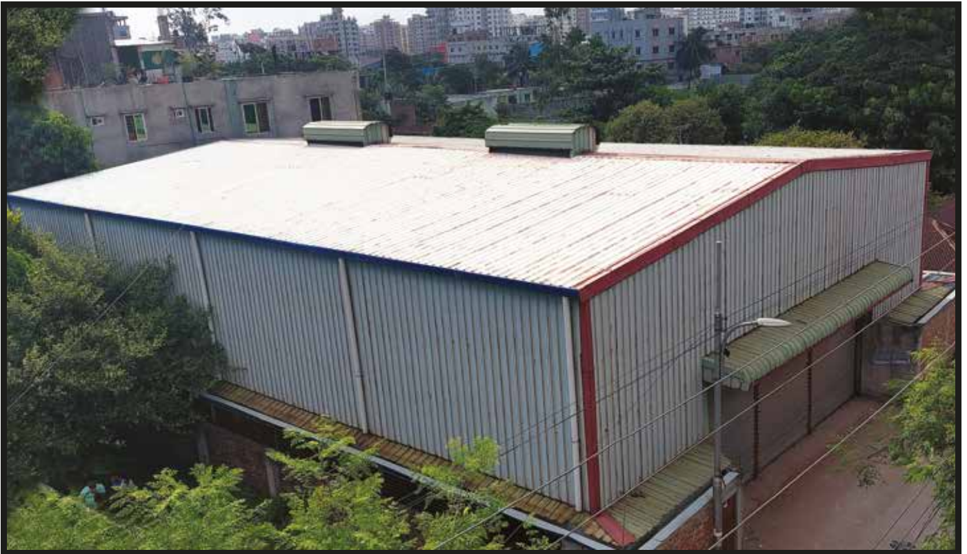
Factory Shed Outer View
