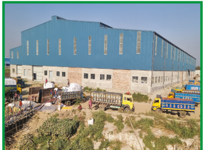
Habib Paper Mills Limited, Rupgonj, Narayanganj.
